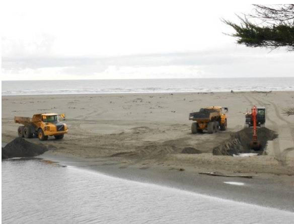
trucks working on the groyne
